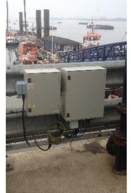
The TideStation Junction Box and wiring loom is fitted for ease of set up and the flexibility to reconfigure/expand the system at a later time.
